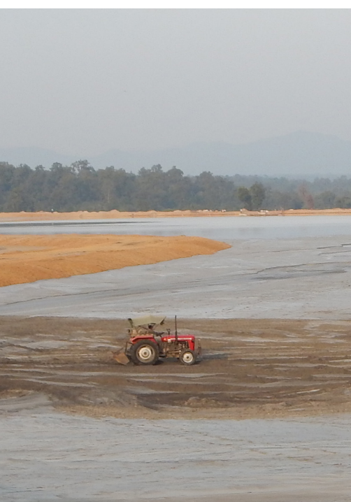
Tractor seen leveling a coal ash pond of the thermal power plant cluster in Korba, Central India.
